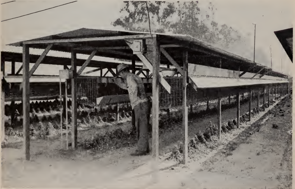
Fig. 39. Two-row single-tier cage hen house. Note overhead sprinklers; also tags on fronts of cages on which a record of the egg production of the bird (or birds) in each cage is kept.
